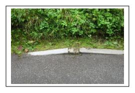
There are five drainage pipes along the spur section and they have all been blocked by tarmac.
